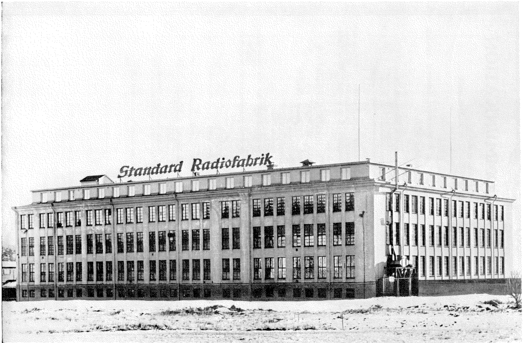
A.-B. Standard Radiofabrik plant in Ulvsunda, Sweden. A wide range of radio equipment is manufactured and includes transmitters and receivers for numerous types of service, vacuum tubes for special purposes, and selenium rectifiers.
